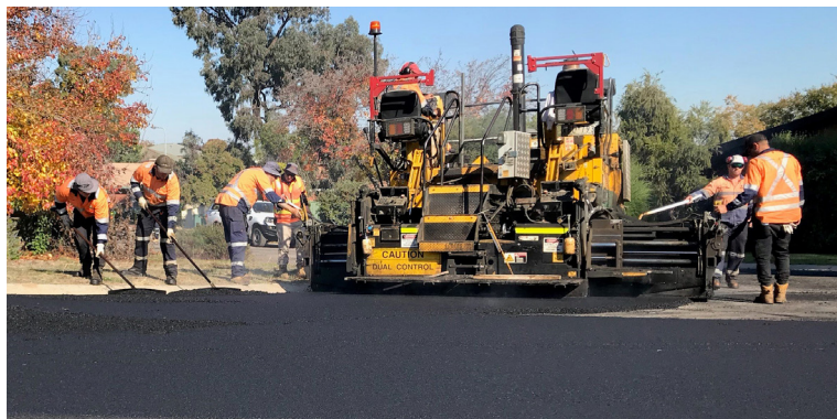
Fume free placement of LTCRA in Bendigo.
