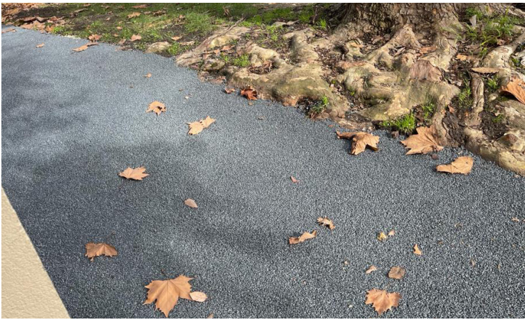
Permeable pavement installed at Banyule City Council, Victoria, 2021
