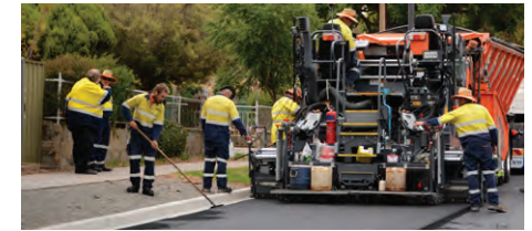
Trial of crumb rubber asphalt in resurfacing of Stanlake Avenue in the City of Mitcham, Adelaide. Approximately 850 used tyres were recycled in this application with the aim to improve road durability.
