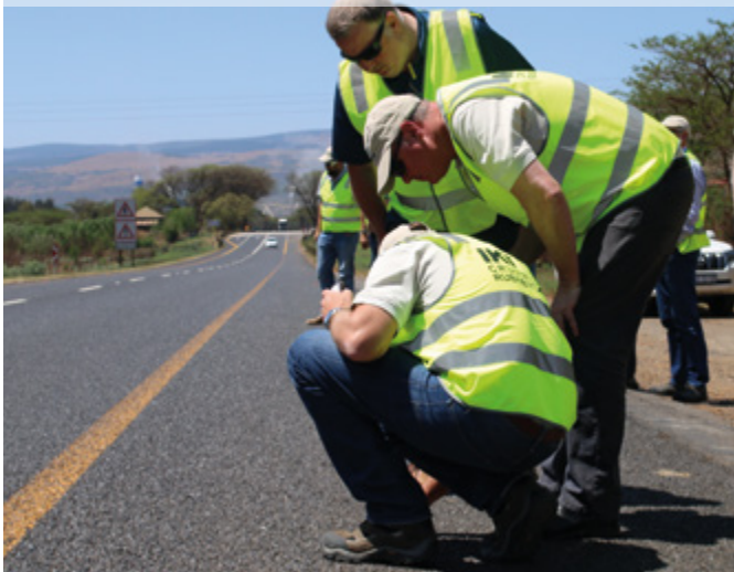
Inspecting road installed with crumb rubber modified asphalt product during South African study tour.
